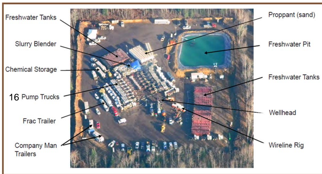
Figure 1: A typical current technology hydraulic fracturing site
