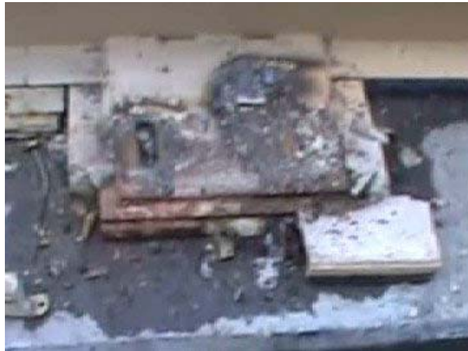
Figure 8: Advanced Corrosion on Various Equipment Support Structures.
