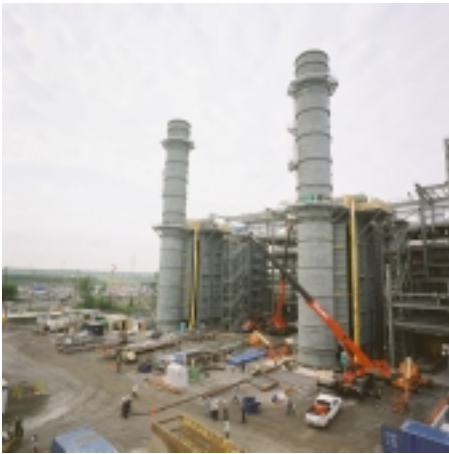
HRSGs Under Construction at Becancour
